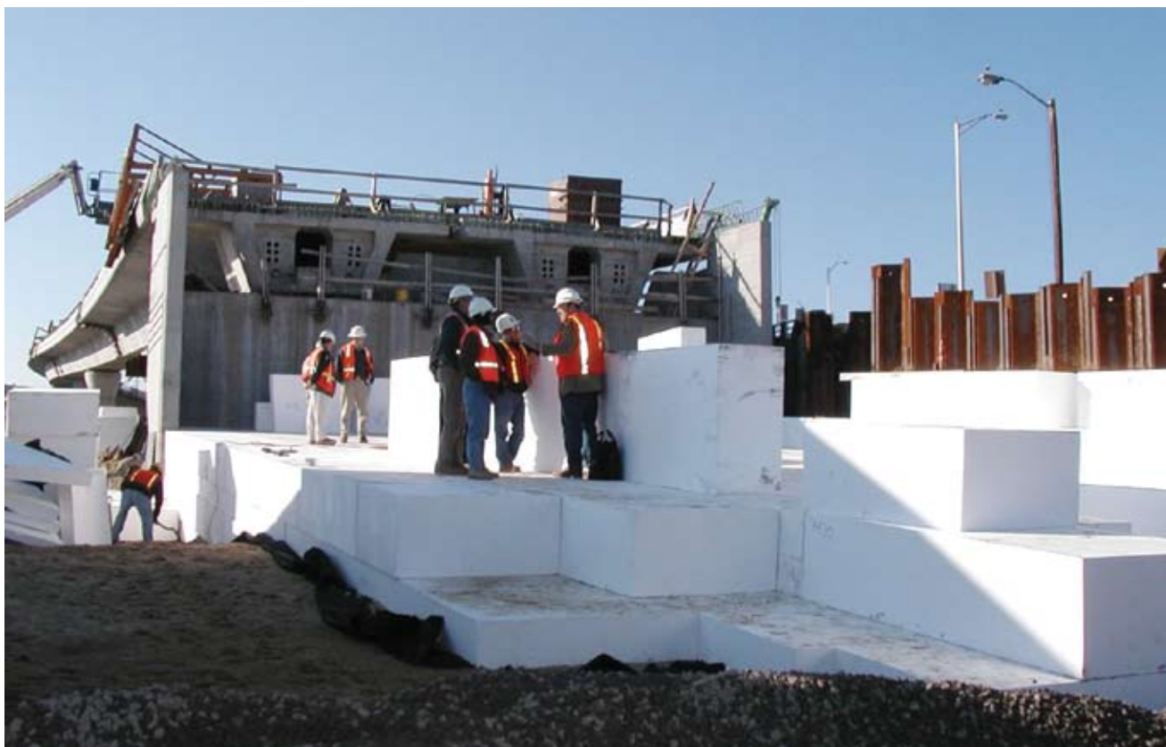
Figure 1. Massachusetts Central Artery/Tunnel embankment fill.
