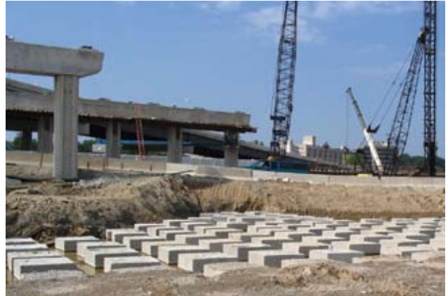
Figure 3. Pile-supported embankment pile caps.
