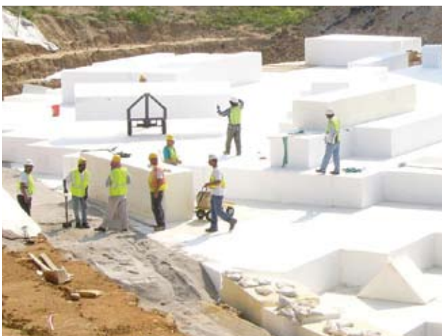
Figure 3. VA Route 1 over I-95 embankment fill.
