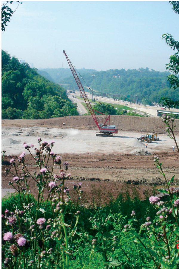
Compaction of the fill material across the building footprint was achieved using a 15-ton weight dropped from 70 feet.
