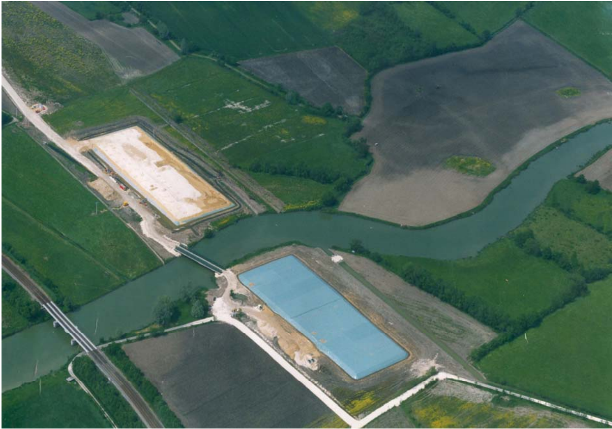
Boutonne River site during vacuum
